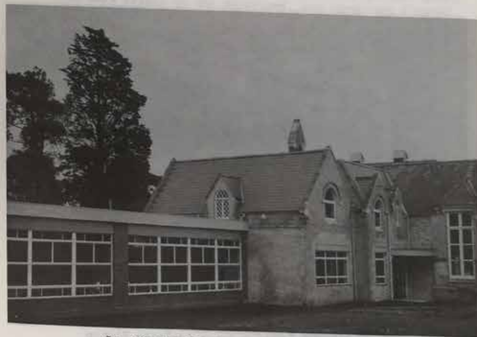
St. Mark's School with modern extension
